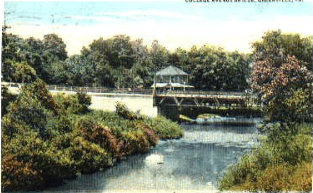
COLLEGE AVENUE BRIDGE, GREENVILLE, PA.
